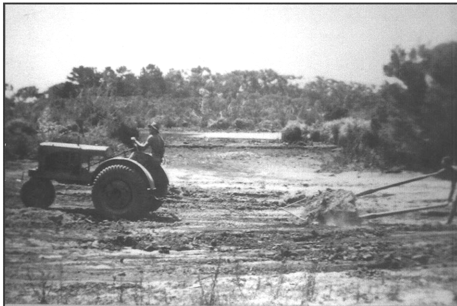
1938 During a dry season, work is carried out on the lagoon.
