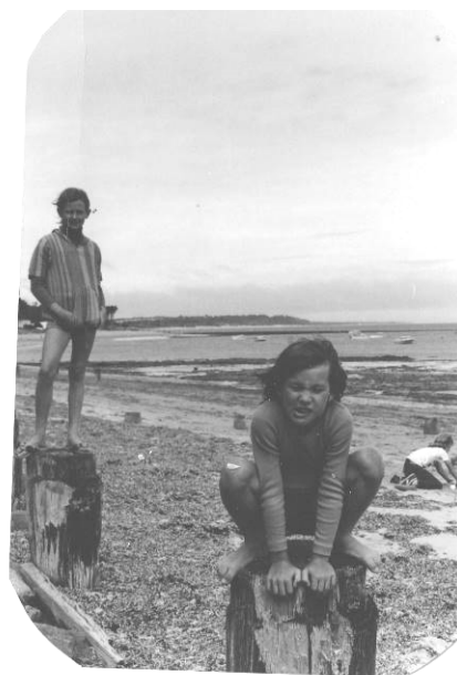
Atop the wooden groynes
